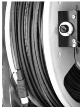
Picture 5: Plug connection on permanently built-in cable drum
